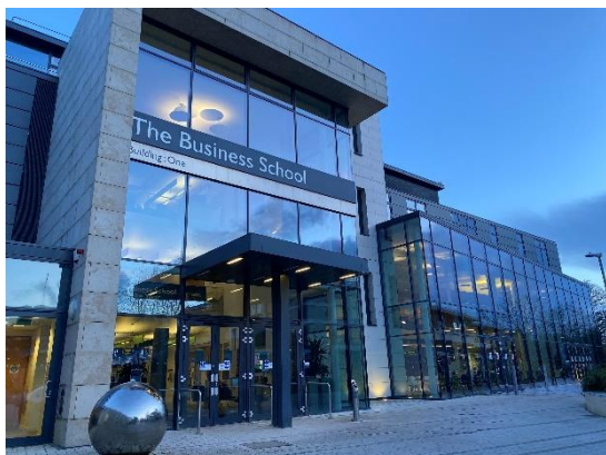
Main building of Exeter Business School
